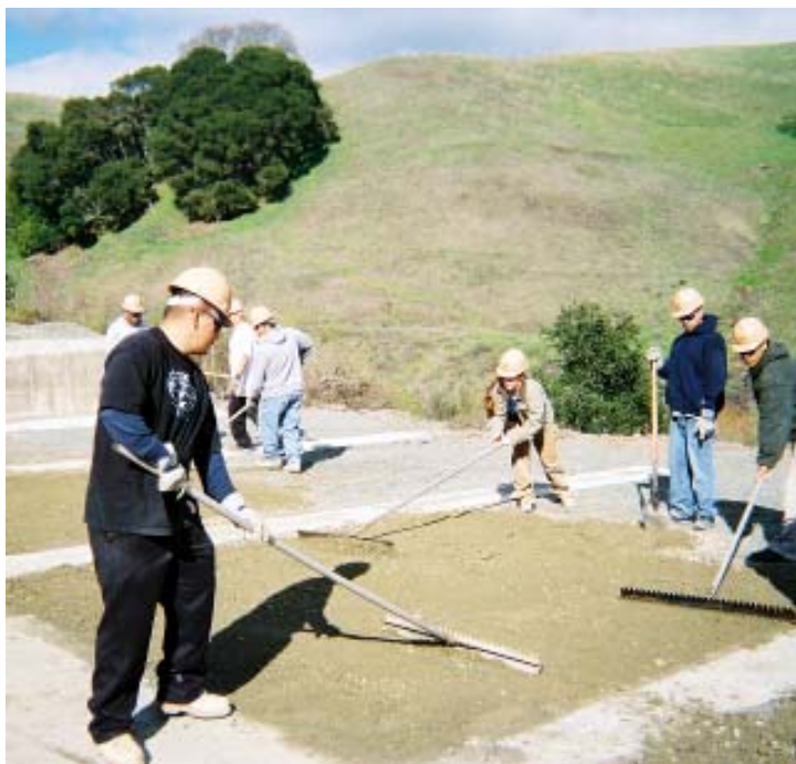
Apprentices practice raking techniques.
